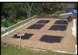
Lay out your ProBase on a firm and level sub base Fill with 10mm round pea gravel
